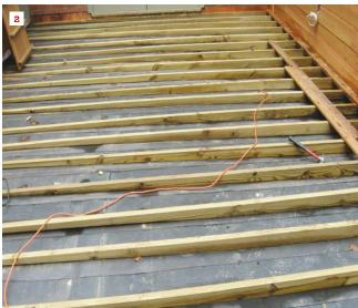
When installing decks over living space, the author adheres to a code-mandated minimum <sup>1</sup>/<sub>4</sub>-inch-per-foot roof slope, which can be achieved by either sloping the roof framing or using a tapered insulation system. While uniformly deep 2-by "floating" sleepers laid across a sloped roof may be installed (1), most clients prefer a level walking surface, so sleepers are typically tapered (2).
