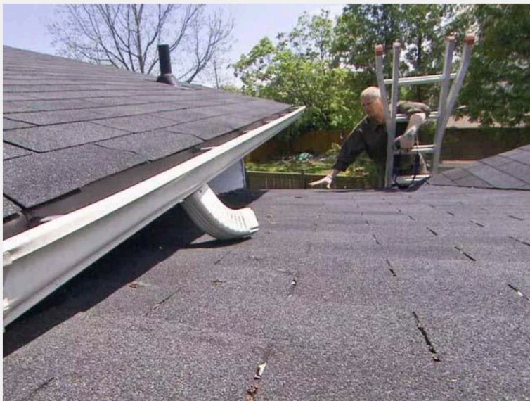
Clean gutters, check for leaks & make sure they're attached securely and check for signs of damage.
