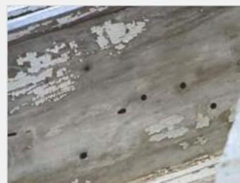
Photo of carpenter bee damage
